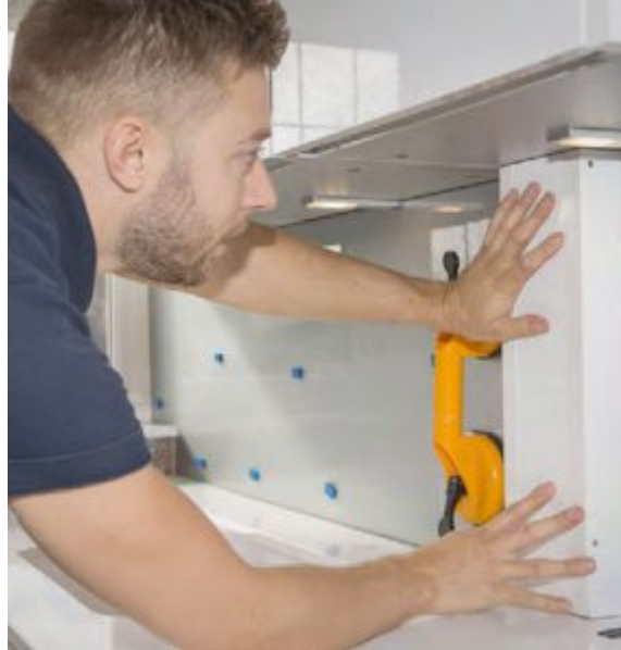
Survey and installation
